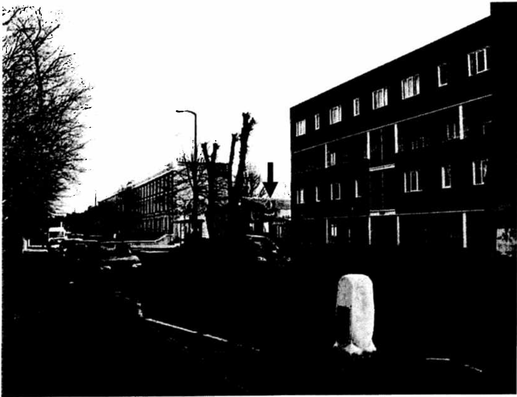
View of former library building and Victoria Park Road (library building denoted by arrow)
