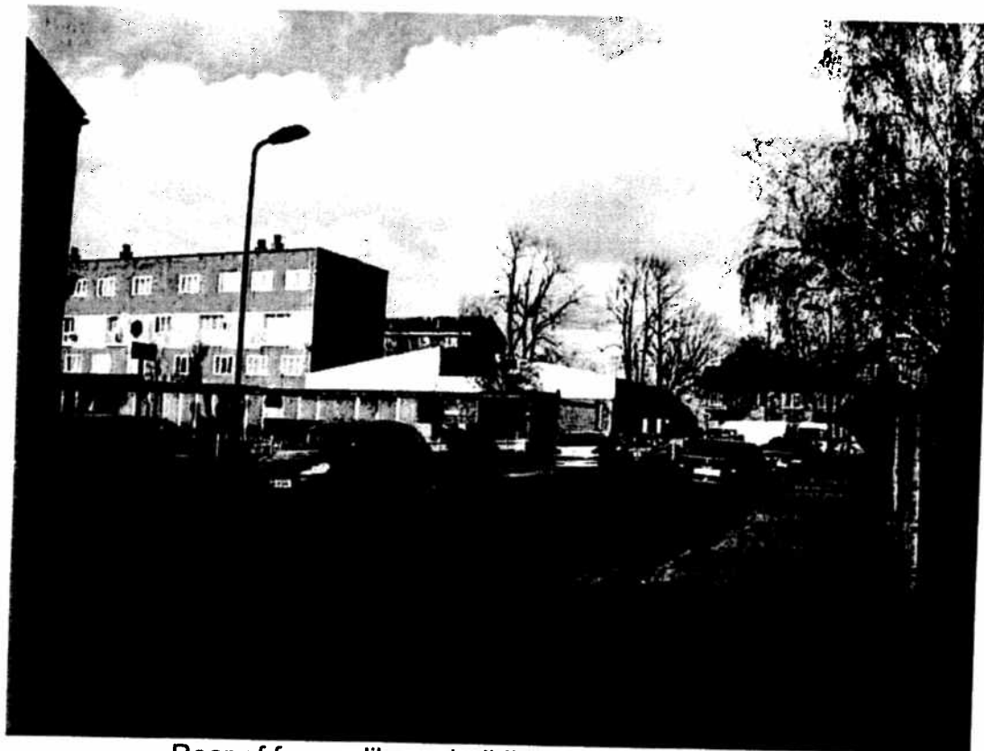
Rear of former library building from Redruth Road
